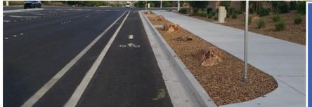
**Buffered Bike Lanes** are visually separated from traffic and/or parking by a striped buffer, but lack any physical separation.
