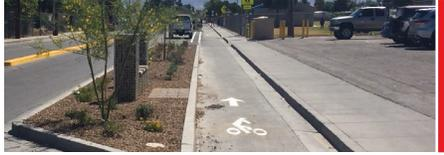
**Separated Bike Lanes** are physically separated from motor vehicle traffic, designed to create the feeling of a trail, but with on-street connectivity.
